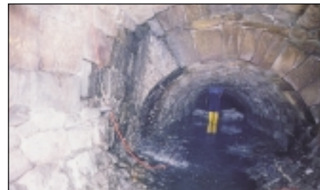
This photo shows the site-constructed temporary pipeline portion of the “flume” operation.
