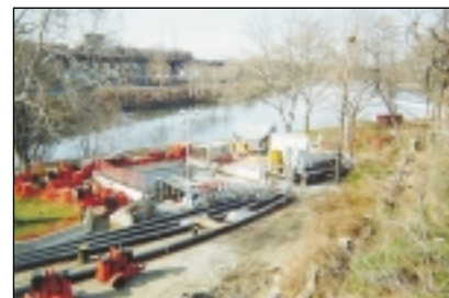
Extensive by-pass operation in Philadelphia, PA
