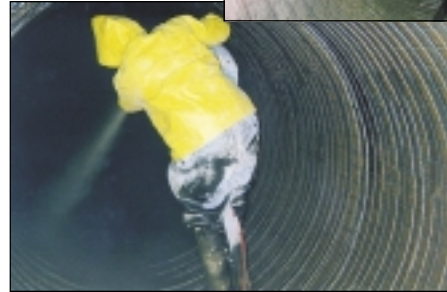
The installation of SewperCoat 2000HS in an insitu concrete trunk line.
