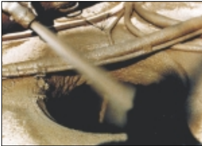
Typical SewperCoat manhole application
