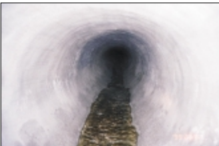
Rehabilitated trunk line in Decatur, IL.
