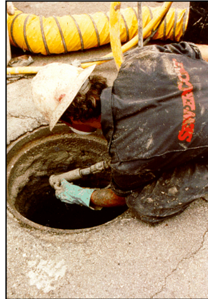
A typical rehabilitation installation...
