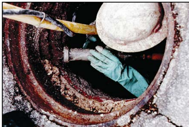
Manhole receiving a SewperCoat® PG installation Rehabilitated brick manhole
