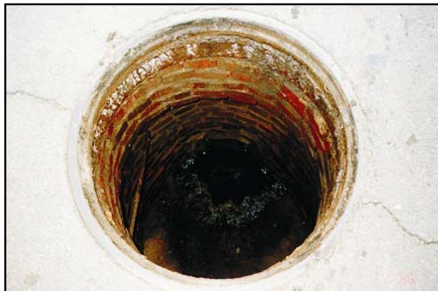
Manhole receiving a SewperCoat® PG installation Rehabilitated brick manhole
